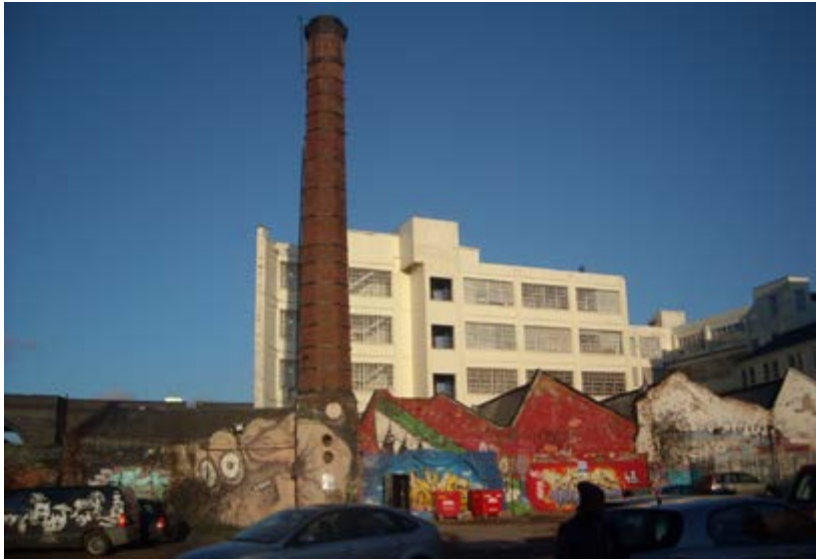
The former Custard Factory, adapted as an arts and media production centre
